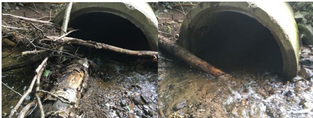
Figure 7 : Before and After photos of debris removal at culvert barrier ELB002.
