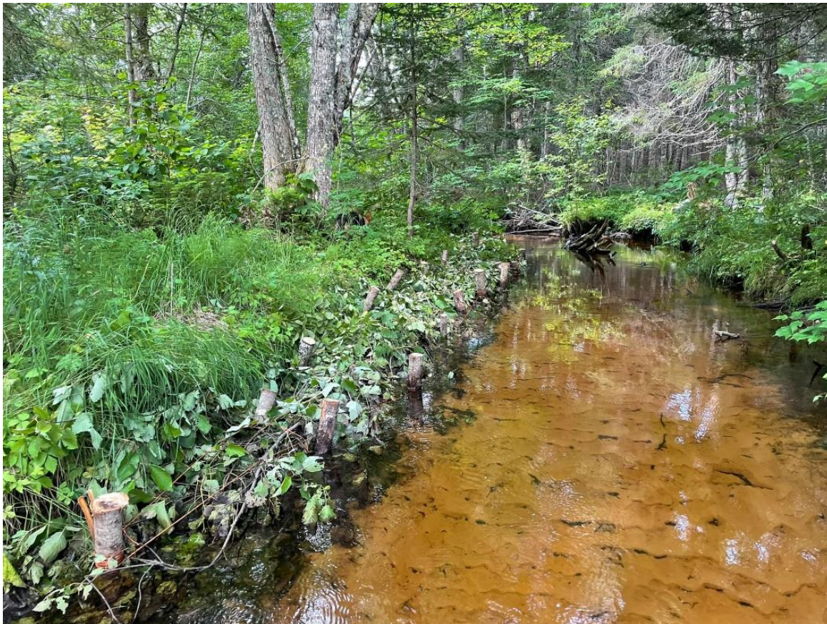
A brush mat built along the south branch of the Morell River to collect access sediment.
