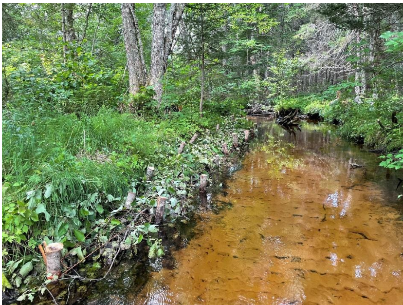
A brush mat built along a section of the south branch with heavy sediment load.
