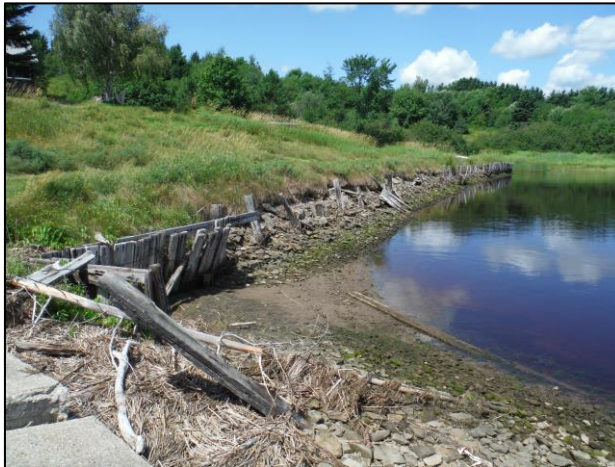
Pre-restoration photo displaying failing creosote wall (2012)
