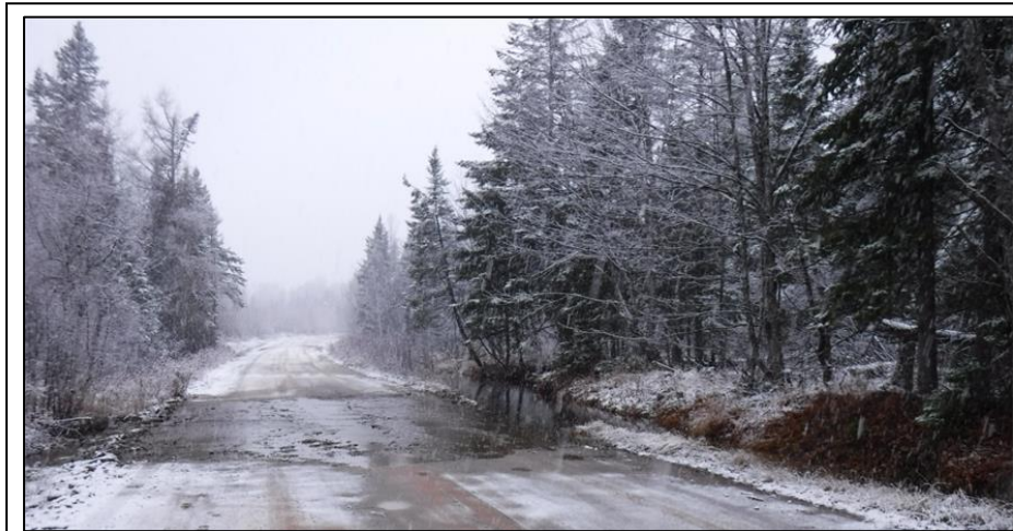
Image above displays Little Beaver Brook flanking culverts and establishing new channel on ch. Desherbiers. This is a significant source of sedimentation into the watercourse
