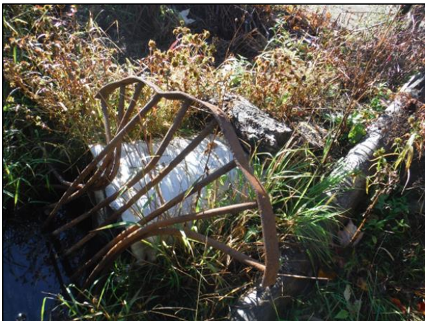
Image above displays inlet of culvert #2 on Beaver Brook. Significant backwatering is observed.
