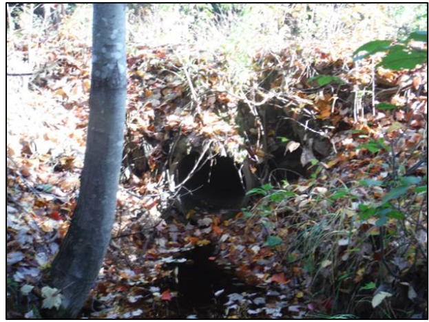
Image above displays outlet of culvert #1 on Beaver Brook. Severe erosion occurring on surrounding culvert, culvert is too short (~10 meters) and should be extended to ~15 meters to allow for proper grading.
