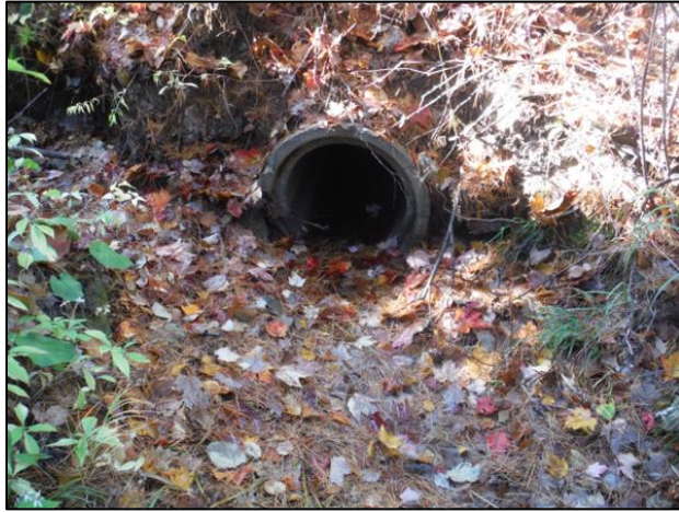
Image above displays inlet of culvert #1 on Beaver Brook. This channel of the stream is usually flowing during high precipitation events. Significant erosion and sedimentation is present due to washouts from roadway.
