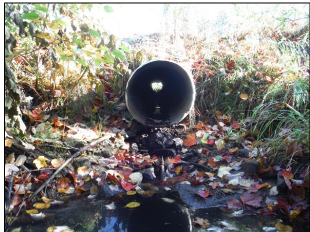
Image above displays outlet of culvert #2 on Beaver Brook. Culvert is perched and broken in middle.
