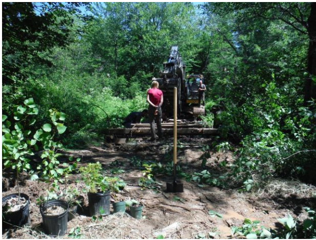
Before photo displaying bridge removal and exposed trail substrate (2018)
