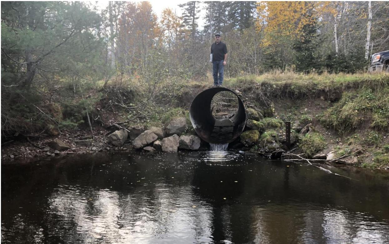
Figure 34: Barrier culvert on MacKinnon Rd on reach 5 ( $61^{\circ}18'16''\text{W}$  ,  $45^{\circ}57'12.9''\text{N}$ ).
