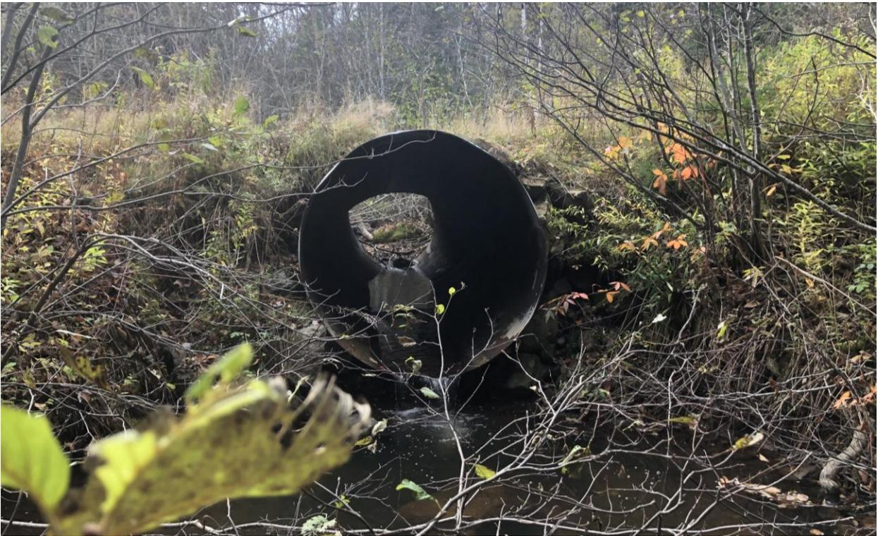
Figure 36: Complete barrier to fish passage on north branch of reach 6 - MacKinnons Rd ( $61^{\circ}17'33.3''\text{W}$ ,  $45^{\circ}57'3.4''\text{N}$ ).
