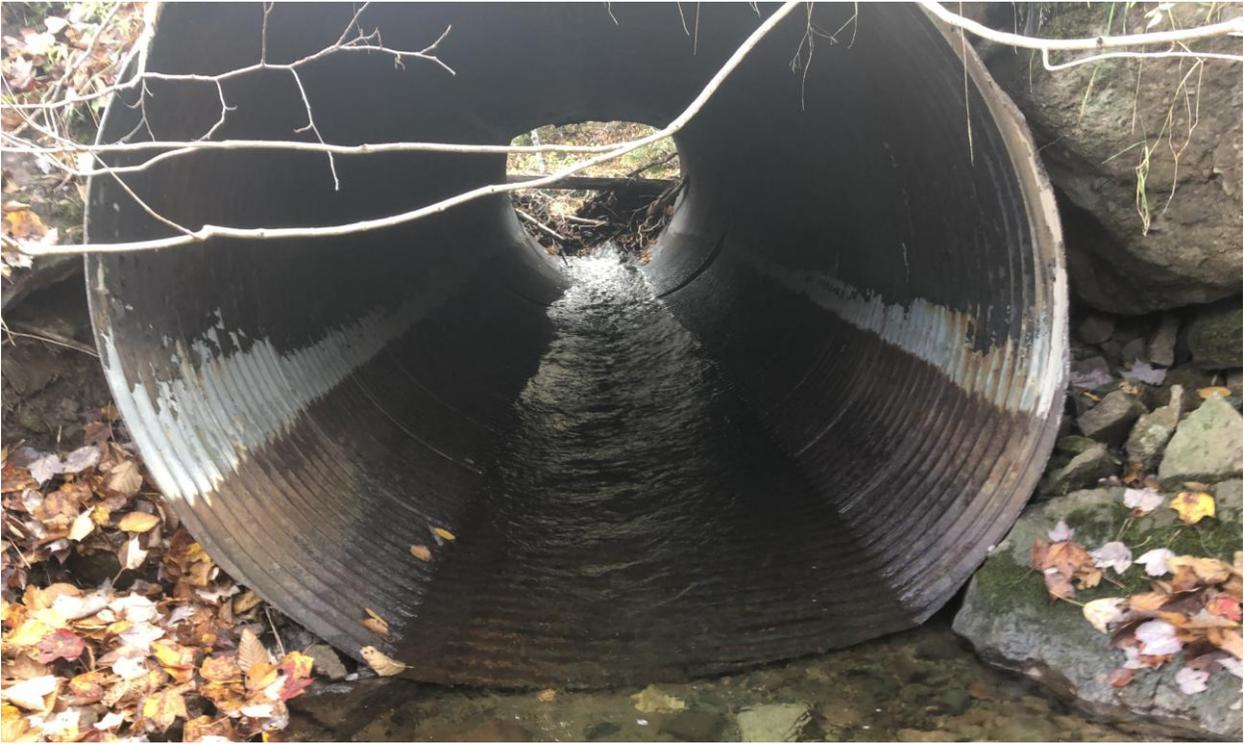
Figure 35: Partial-to-complete fish passage barrier on reach 6 MacKinnon Rd crossing ( $61^{\circ}17'38.2''\text{W}$ ,  $45^{\circ}56'60''\text{N}$ ).
