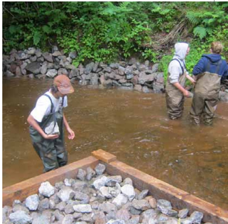
Installing deflector structure Photo: ASCF
