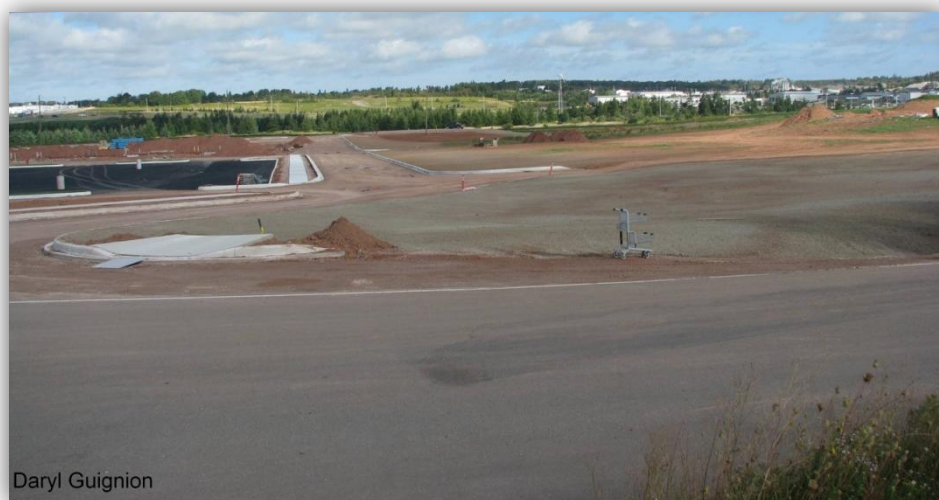
Figure 8.8 Impervious surfaces and exposed piles of soil combine to create serious soil erosion issues during rain events in Charlottetown
