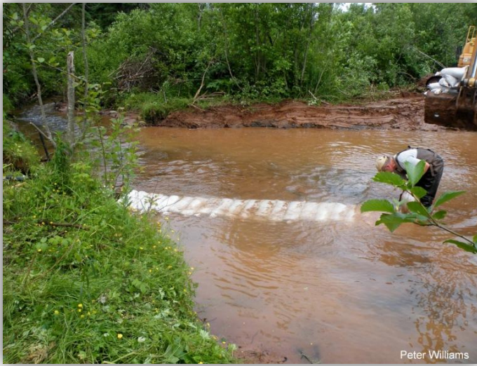
Figure 8.15 Construction of a sandbag barrier to close off the original stream channel and divert stream flow into the bypass pond (shown here on West River)
