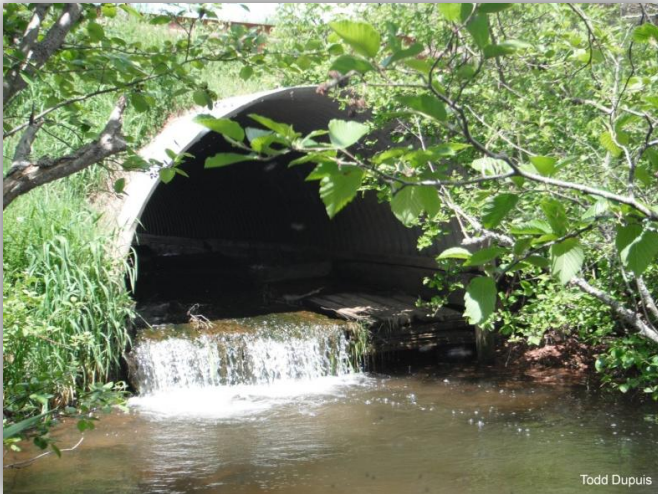
Figure 4.8 Perched culvert, Clyde River
