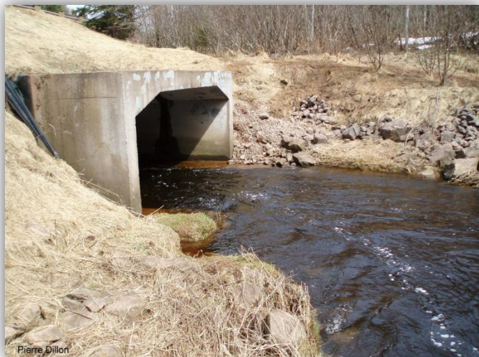
Figure 13.10 Prefabricated, natural bottom culvert installation on Lennox Island
