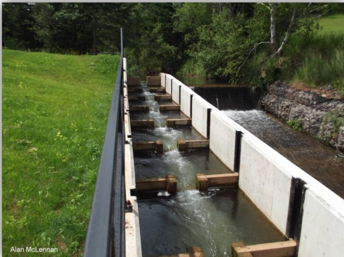
Figure 13.13 Newly constructed fish ladder at Parsons Pond on Granville Creek
