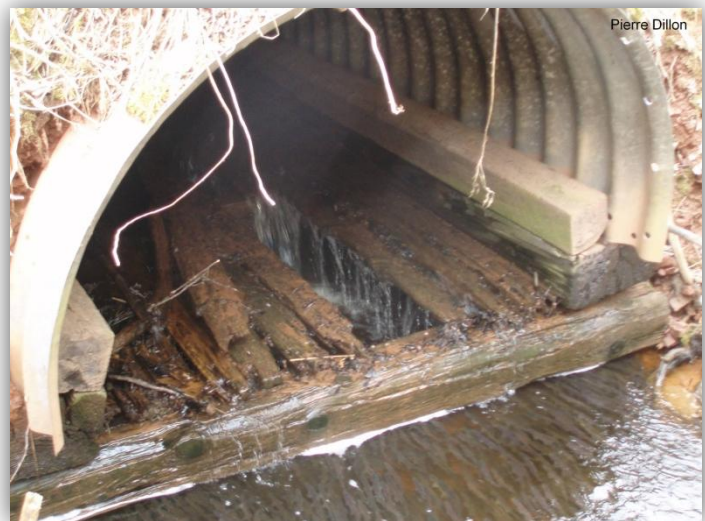
Figure 13.4 Rotten flooring in culvert on Joey's Road, blocking passage of rainbow smelt
