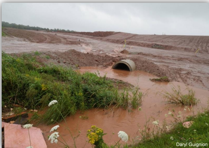
Figure 8.7 Traditional storm water infrastructure was inadequate when an intense rain event coincided with the construction of a new mall in Charlottetown, summer 2011
