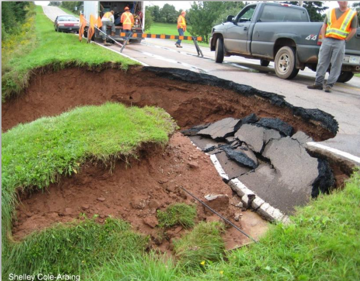
Figure 3.27 Culvert collapse on Brackley Point Rd (top) and flooding of Lower Malpeque Rd (bottom) during an extreme rain event, September 2008
