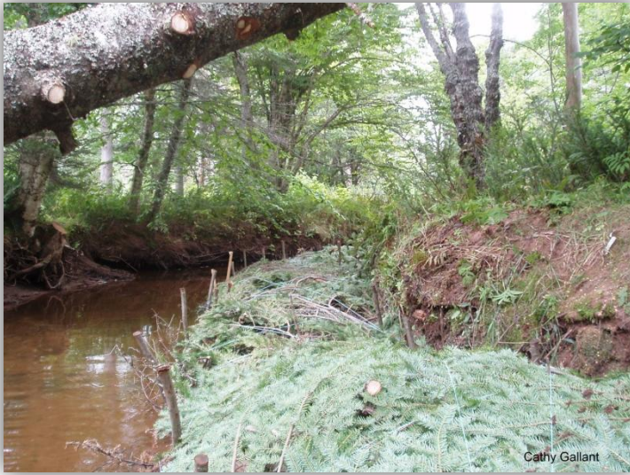
Figure 10.1 Completed brushmat on the Little Trout River
