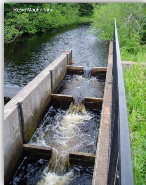
Figure 13.14 Pool and weir fish ladder on the Vernon River
