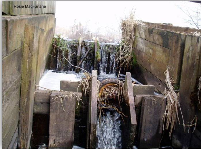
Figure 13.19 Island fish ladder blocked with trash
