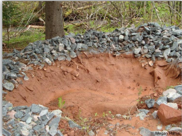
Figure 8.6 Trap on Ross Road (Brookvale) intercepts sediment running down the road before it can reach the river (background)
