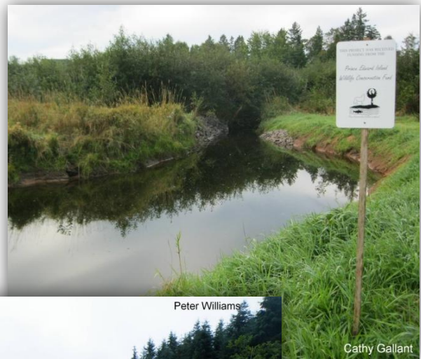
Figure 8.13 Two examples of bypass sediment ponds: the original stream channel is visible at the point of granite armouring (top right, Trout River) and behind the partially completed sandbag barrier (bottom left, West River)
