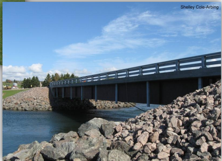
Figure 13.12 Two renovated bridge structures on the Trout River, Tyne Valley (top) and West River (bottom), showing concrete or rock bank reinforcements and no in-stream piers
