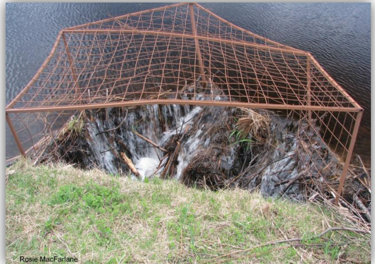
Figure 3.19 Drop inlet culvert with beaver exclosure cage, catching debris and blocking fish passage
