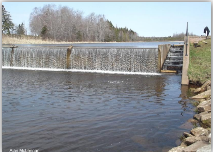
Figure 14.3 Hunter's Pond in Baltic (top) is contained behind an earthen berm with a run-around bypass channel that does not block fish passage, whereas Livingstons Pond on Big Pierre Jacques River (bottom) has a concrete dam structure with a finite lifetime
