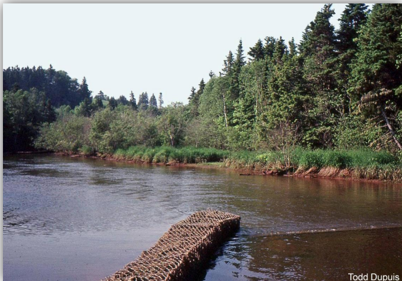
Figure 12.7 Older style gabion basket deflector just below the head-of-tide, West River
