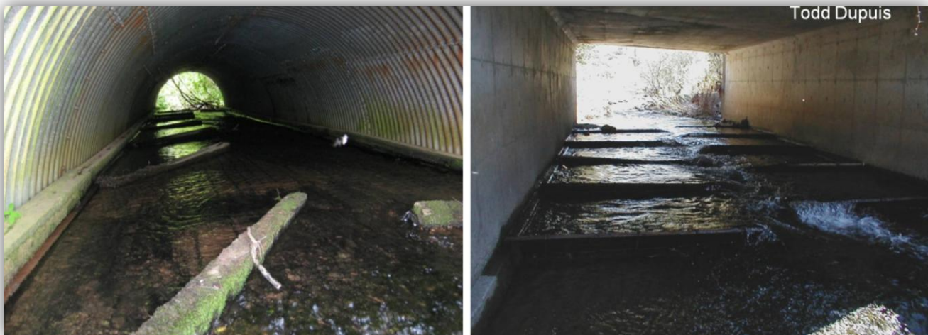
Figure 13.9 Baffles set on the diagonal (left) or perpendicular (right) to the culvert wall
