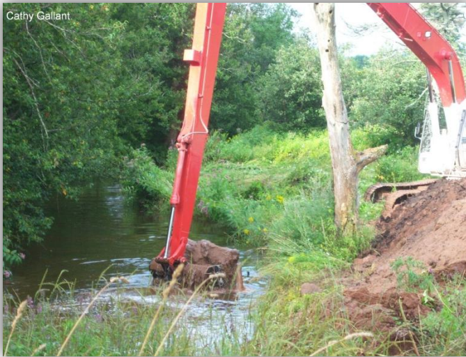
Figure 8.11 Hymac excavator removing sediment from the in-stream trap shown in previous figure (Tyne Valley)
