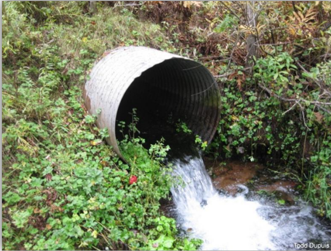
Figure 13.1 Perched culvert with no access for fish from downstream
