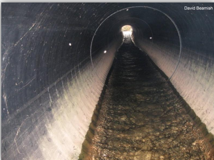
Figure 13.2 Plastic culvert on the West River that is too long and smooth to allow effective fish passage (velocity barrier)
