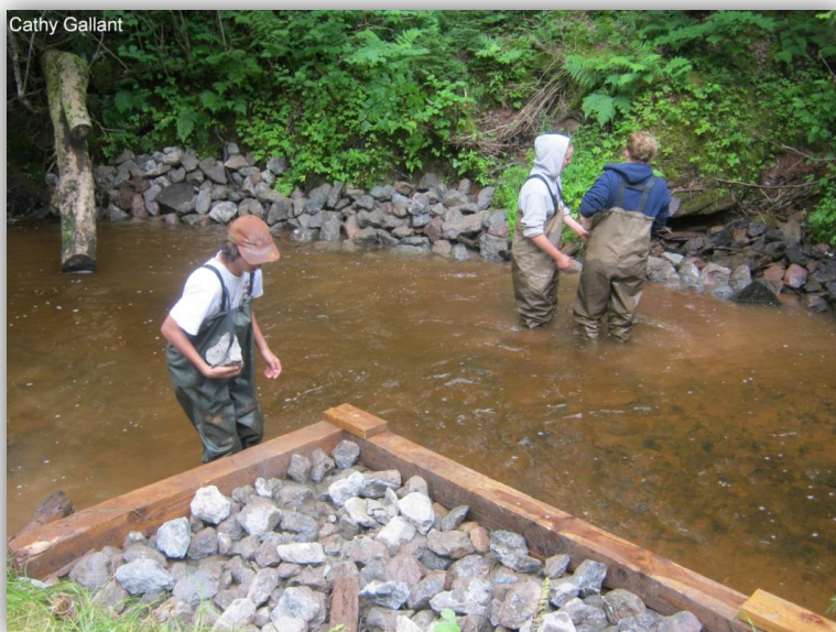
Figure 12.2 Wing deflector construction, Little Trout River
