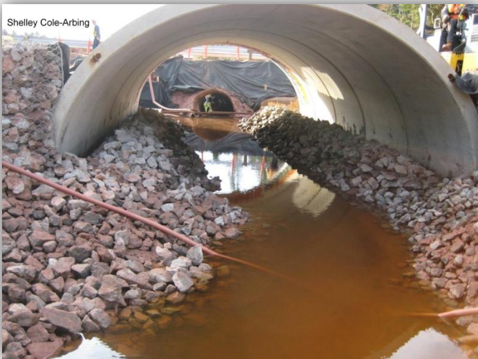
Figure 13.10 Prefabricated, natural bottom culvert installation on Lennox Island
