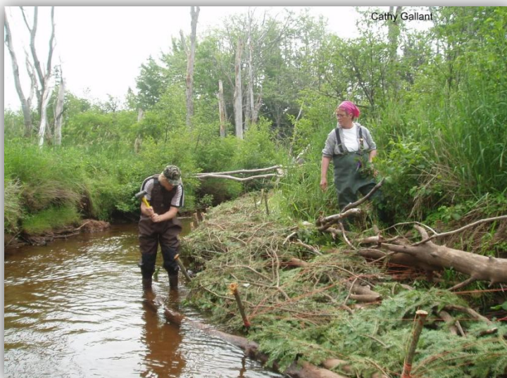
Figure 8.9 Brush mat construction around a point bar in the Little Trout River
