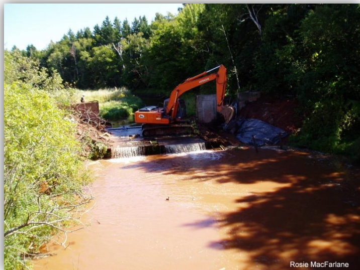
Figure 14.7 Decommissioning of Breadalbane Pond on the Dunk River. Sediment was removed from the stream bed upstream from the dam during the decommissioning process
