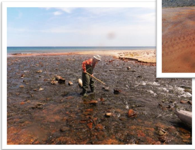
Raking to maintain deeper channel
