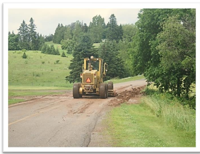
Runoff from potato fields in Grahams Road, July 2018 (above left). A road grader was needed to remove soil from the road (above right)
