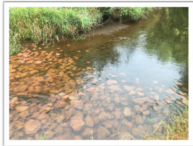
Cobble added to stream bottom in Trout River (Coleman)
