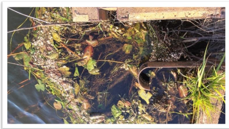
Fish ladder at Robinsons Pond clogged with aquatic vegetation
