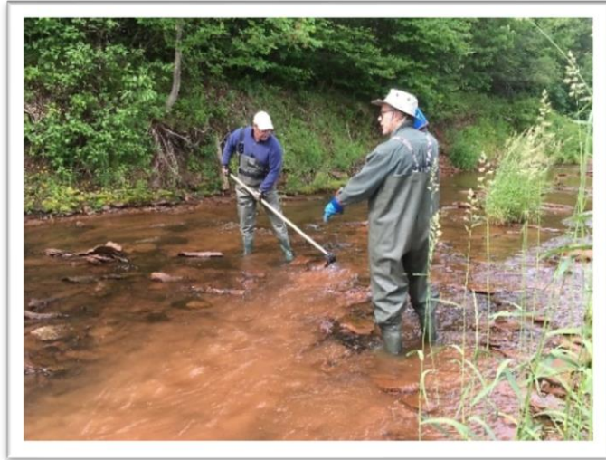
Clam rakes can be used to temporarily excavate a defined channel to improve passage for adult salmon on Cains Brook
