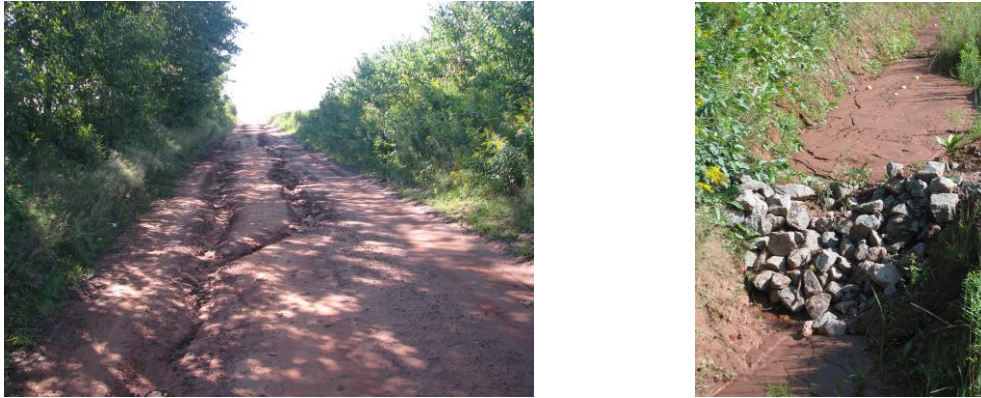
Figure 6. Clay roads are prone to erosion and check dams must be cleaned regularly.
