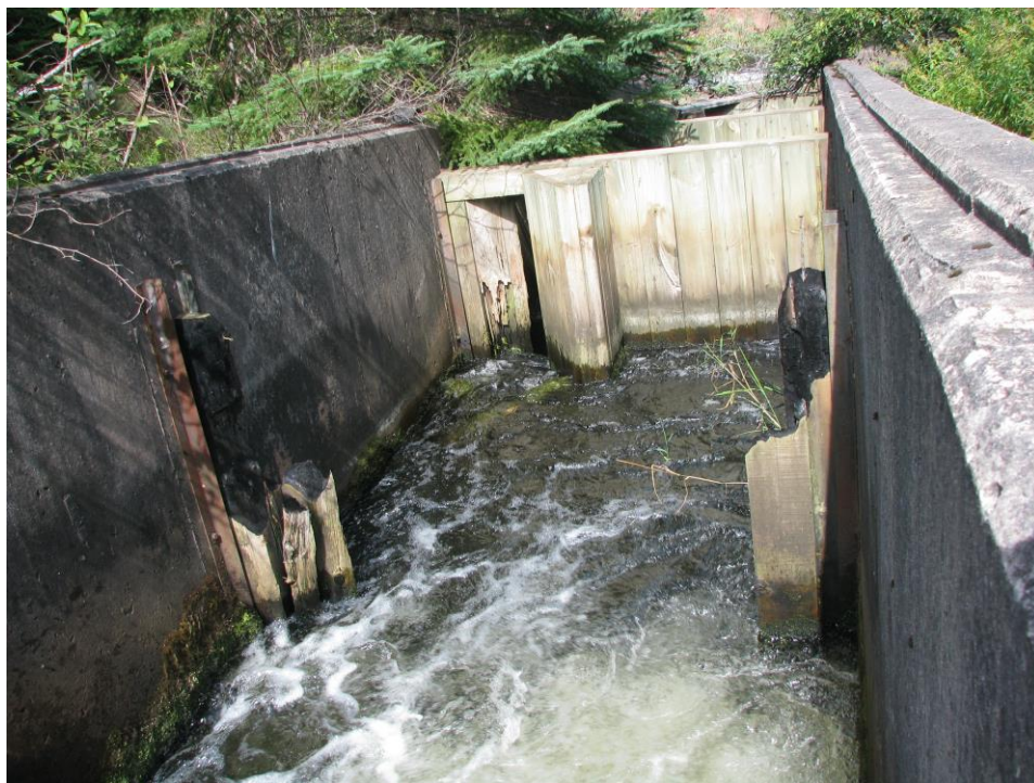
Figure 122. A burned-out cell in the fishway at Maritime Electric Pond on the Valleyfield River.
