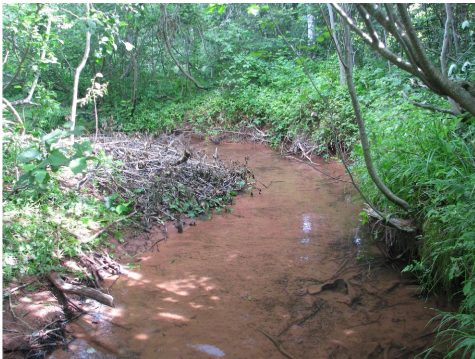
Figure 50. Quinns Brook, downstream from Carraghers Pond. Brush mats are positioned to consolidate sediment and deepen the stream channel.
