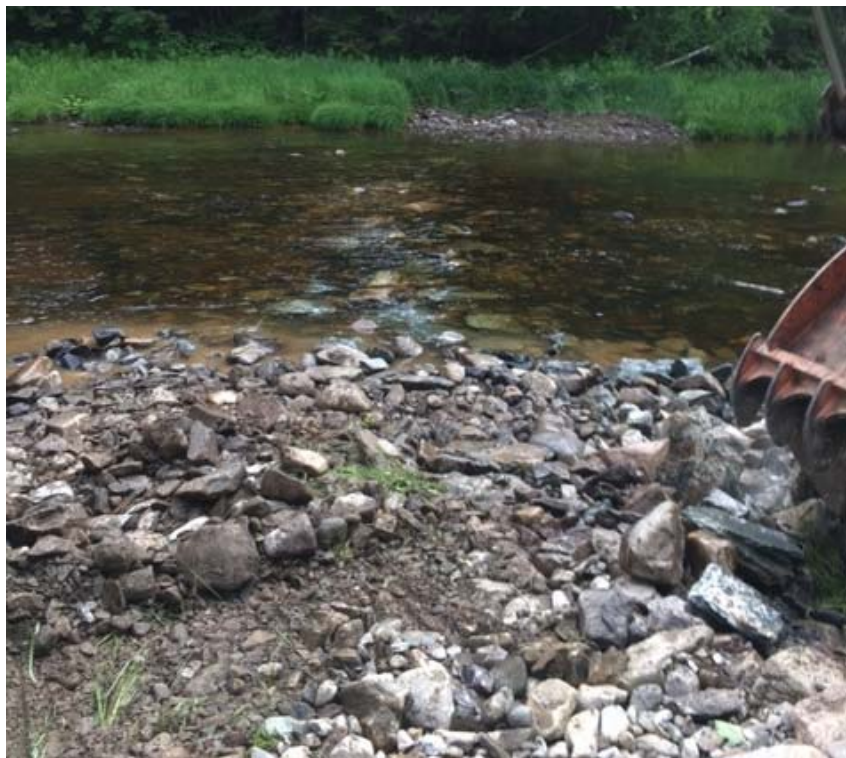
Figure 28: Site 6, structure 6.09 during construction.
