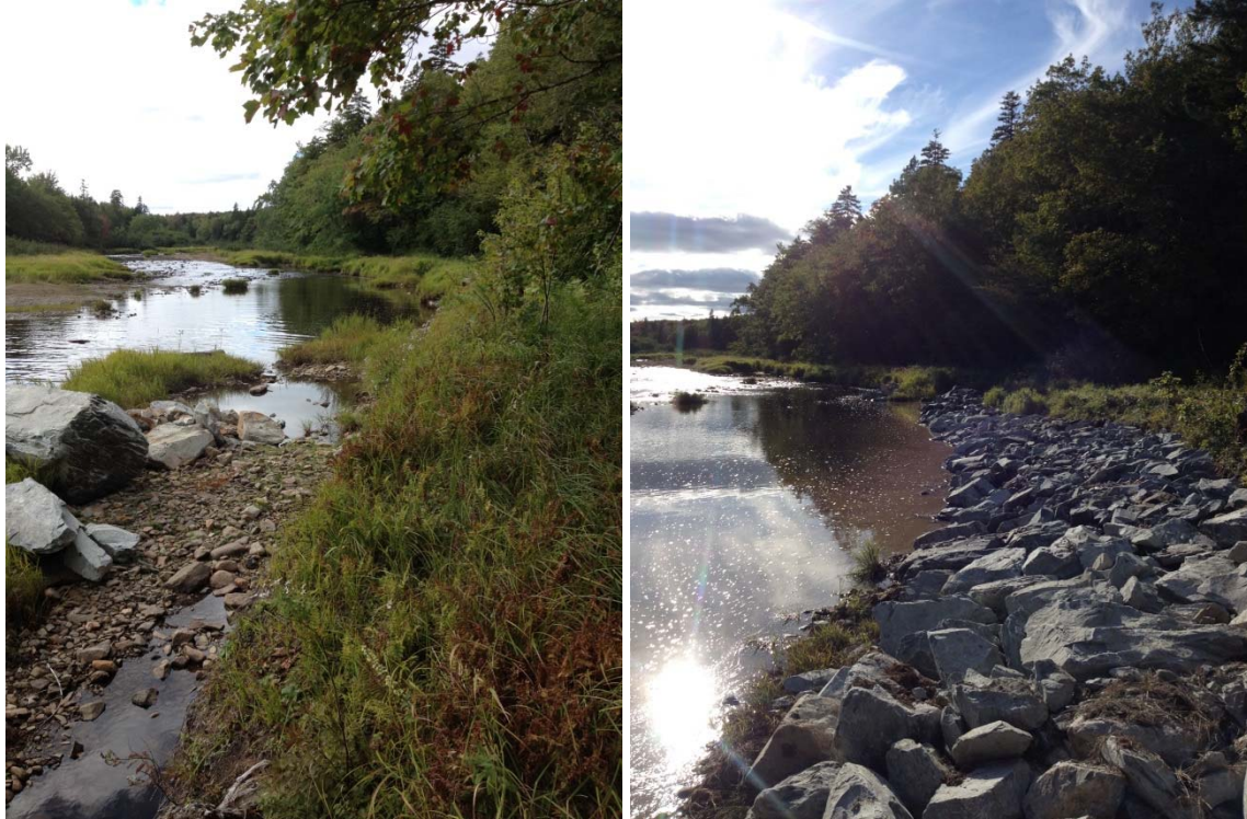
Figure 26: A) Before shot of the pool below sill 2 at Site 5 (structure 5.5). B) This is the bank work below sill two (structures 5.5 to 5.7). Note the 4:1 slope on the bank instead of the normal 2:1 slope. This will assist in the planting of native trees and grasses later.
