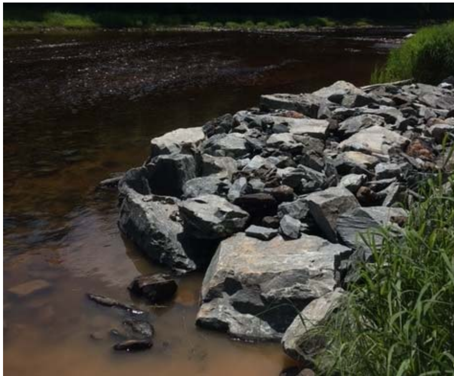
Figure 32: Site 6, Structure 13. Rock deflector
