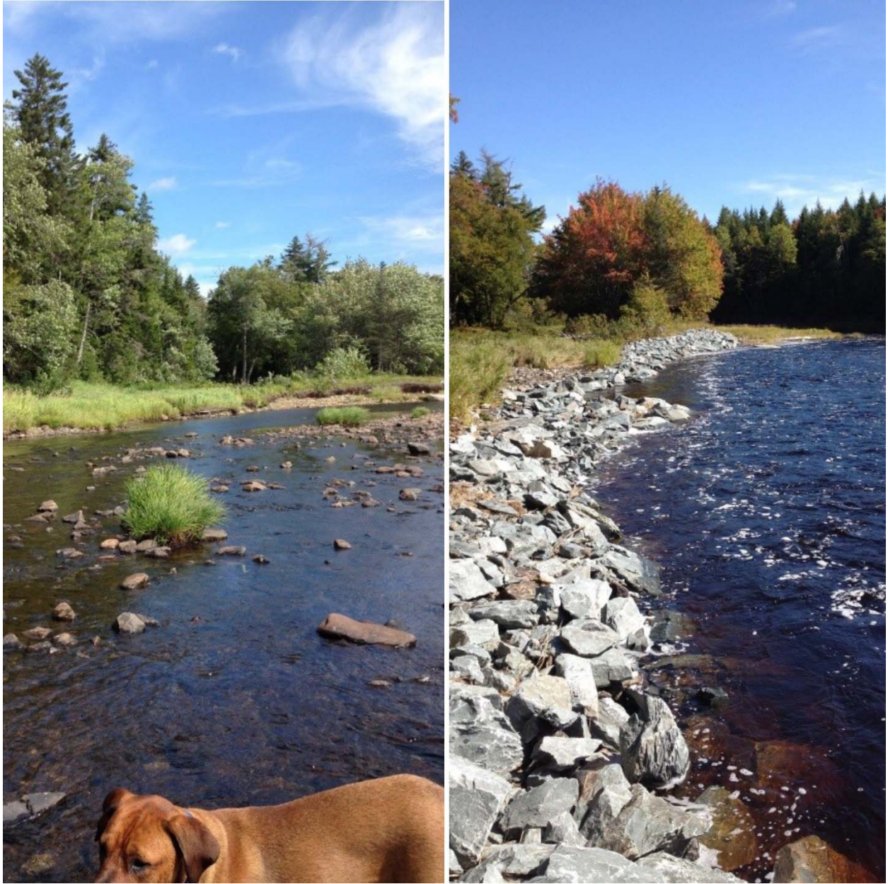
Figure 25: Before and After, armour rock Site 5.
