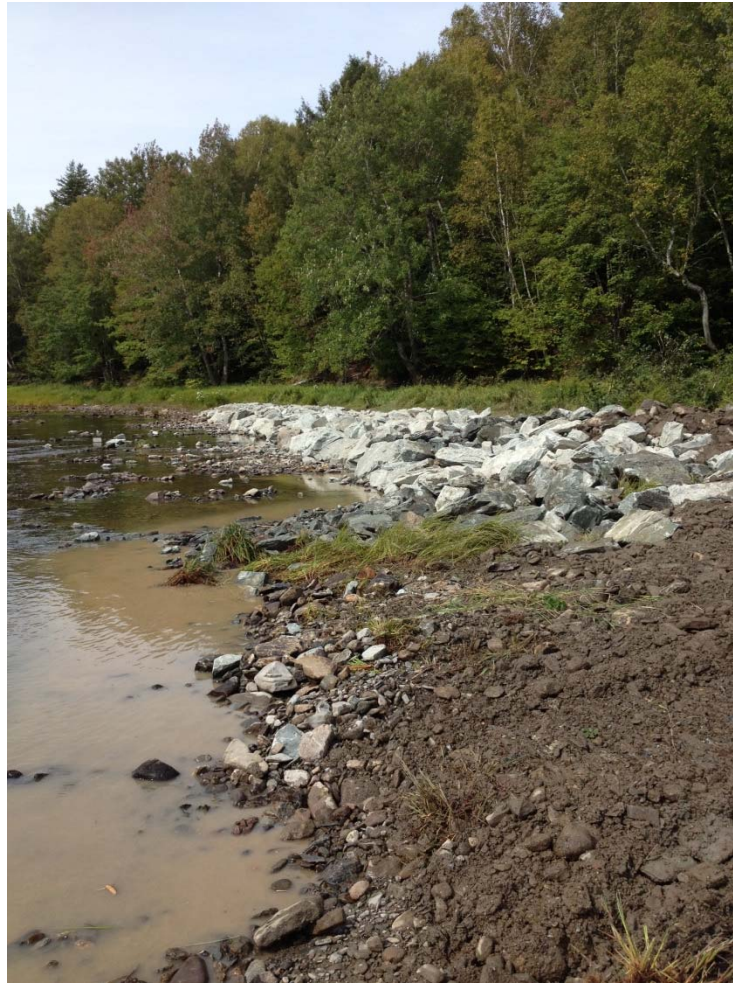
Figure 17: Bank protection installed at Site 5.
