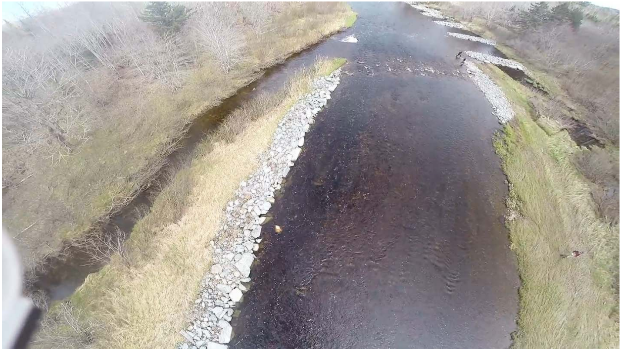
Figure 19: Aerial photograph of armour rock bank.
