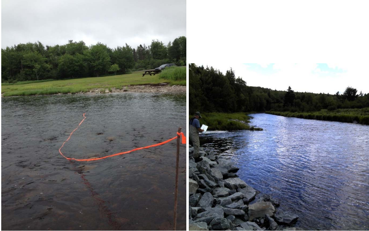
Figure 24. A) Before photo where sill is to be constructed and bank protection is needed (looking at the right bank, facing downstream). B) After photo looking upstream at sill and bank protection.
